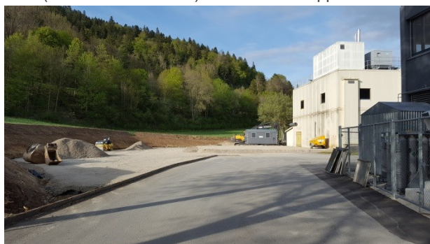
View of the actual construction status
