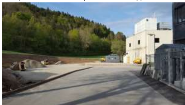
View of the actual construction status
